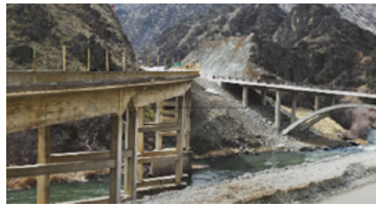
Old Klamath River Bridge (left) with the new bridge in the background (right).
