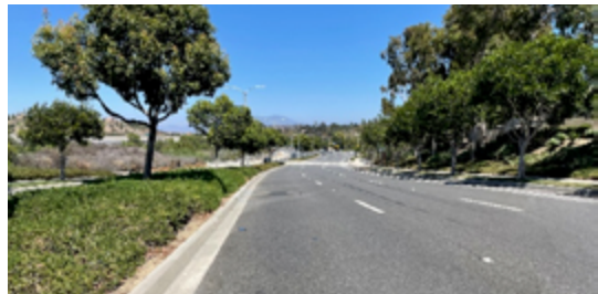
After: Bonita Canyon Drive and Ford Road Pavement Rehabilitation Project.
