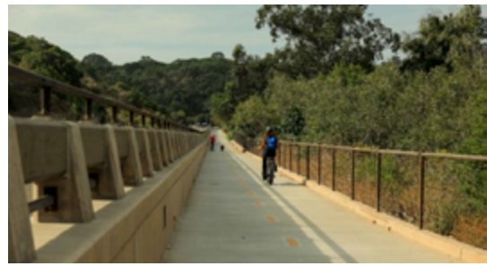
The Las Positas Multi-Use Path built a separate space for bicyclists and pedestrians along a high-speed road with narrow shoulders.
