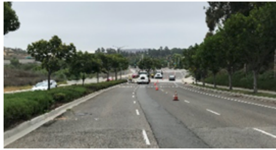
Before: Bonita Canyon Drive and Ford Road Pavement Rehabilitation Project.
