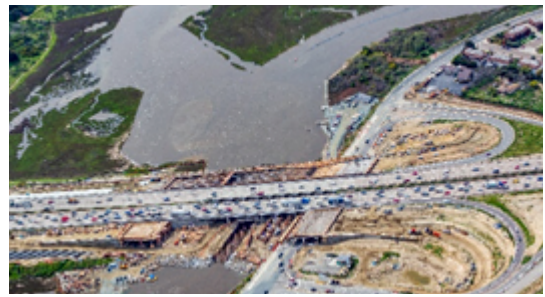
The San Elijo Highway Bridge under construction, in San Diego County.
