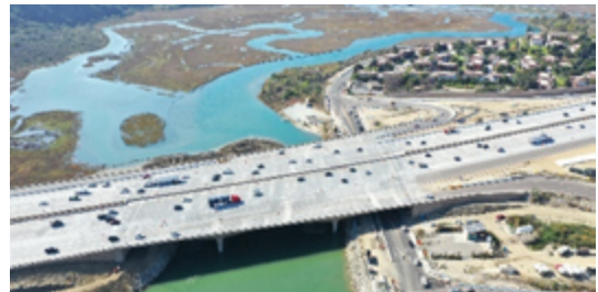
The San Elijo Highway Bridge after construction is complete, with both high-occupancy vehicle lanes open.
