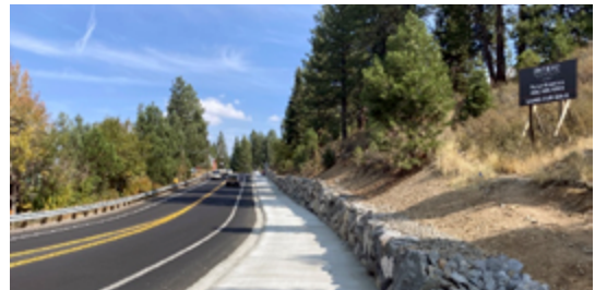
After: Legacy Trail-Brockway Road Multi-Use Trail Connection
