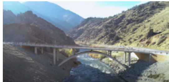
New Klamath River Bridge completed in May 2022.
