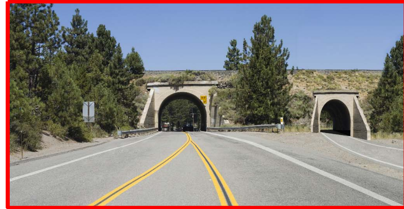
NORTHBOUND LOOKING TOWARD DEERFIELD DRIVE
