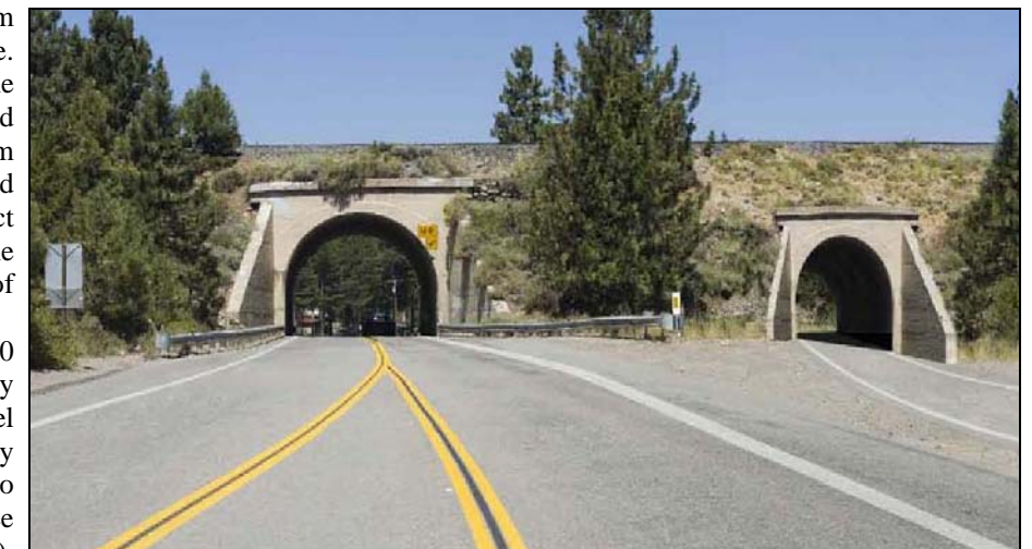
Proposed pedestrian tunnel (on right) looking north on SR 89 at Truckee's "Mousehole"
