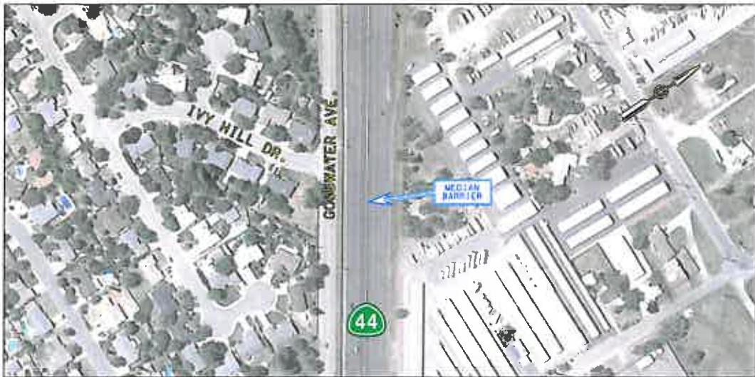
EXAMPLE OF AN EXISTING 36' MEDIAN HIGHWAY 44 IN SHASTA COUNTY
