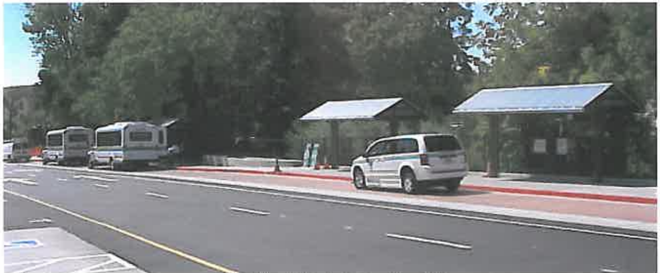
Tinloy Street Transit Transfer Center in Grass Valley
