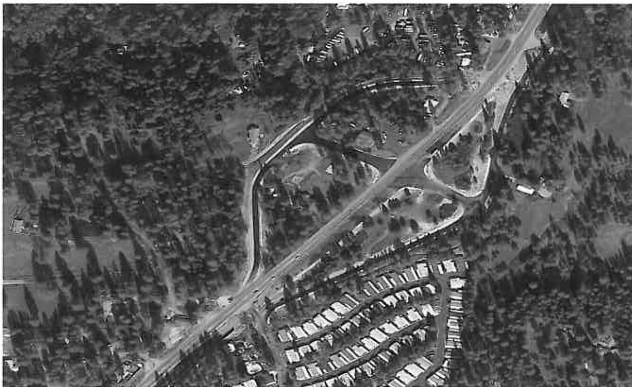
Aerial view of the SR 49 / La Barr Meadows Road Widening Project with Frontage Roads
