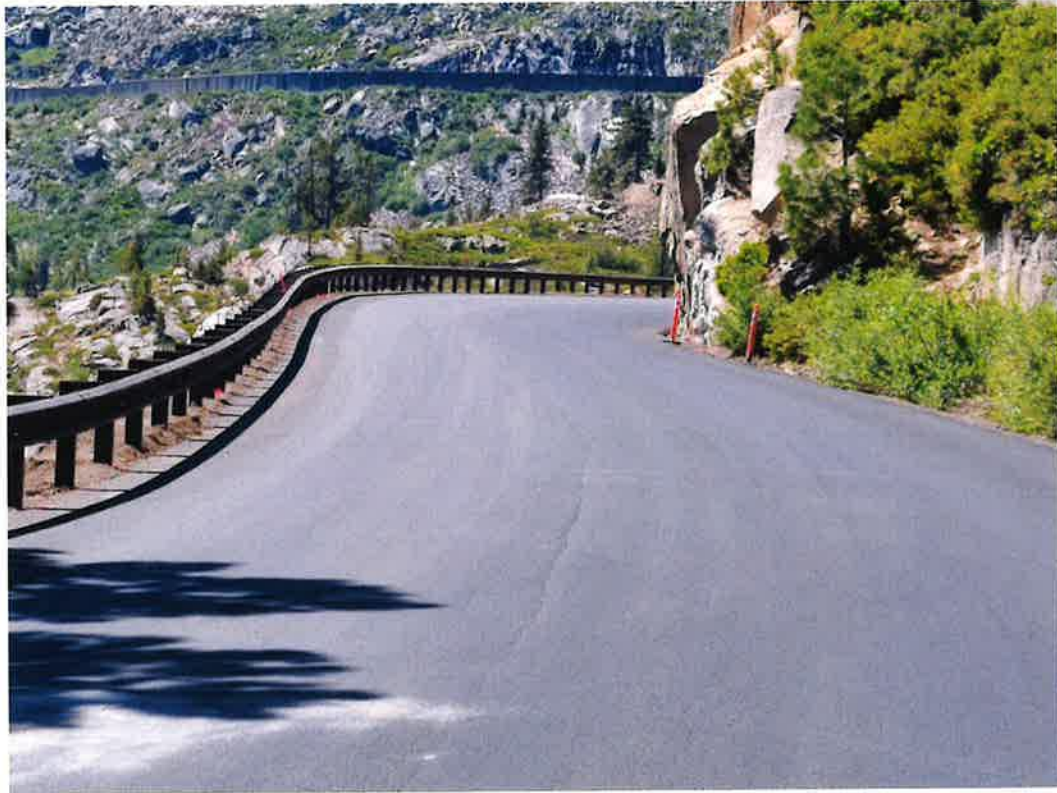
Widening Donner Pass Road
