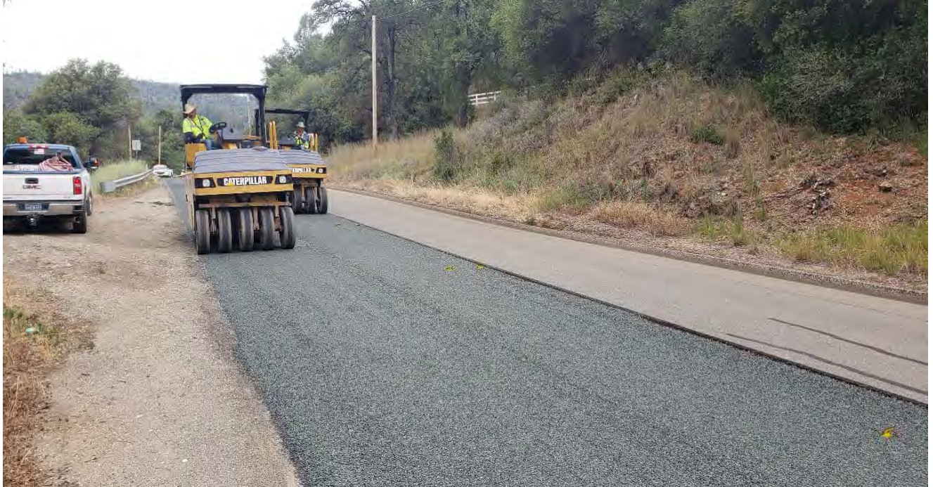
Placing chip seal in Alta Sierra
