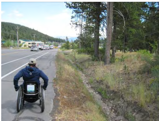
Sidewalks are missing on key segments of Donner Pass Road
