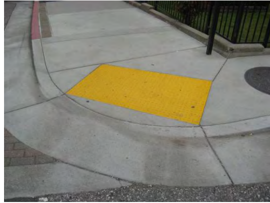
Curb ramps make crosswalks and sidewalks accessible for wheelchairs, strollers, and bikes; the yellow "truncated domes" alert blind and vision-impaired pedestrians as they approach a street
