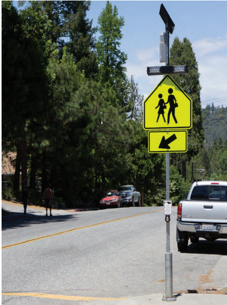
Rectangular rapid flashing beacon, Zion Street, Nevada City
